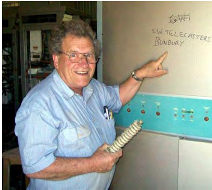
Ian inspects an old transmitter cabinet belonging to his old employer, Southwest Telecasters of Bunbury, now GWN.
